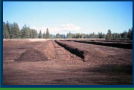
Windrow Composting Facility
